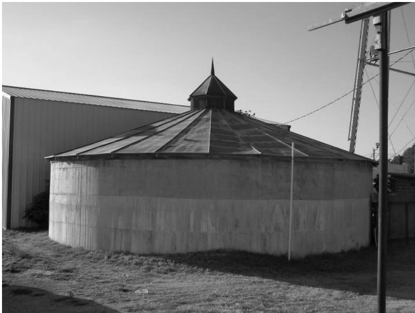
Figure 12.1. Old cement cistern utilized for decades to store water.
