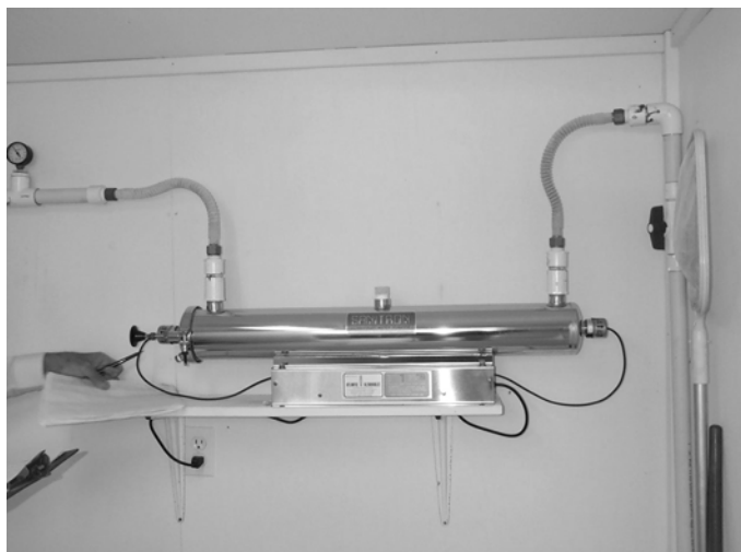
Figure 16.18. Flexible connections on a UV device make installation easy and quick.
