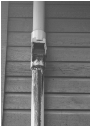
Figure 17.1. An unattended leaf diverter on a downspout.
