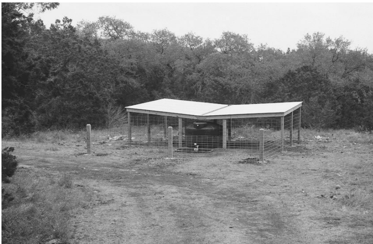
Figure 2.2. A water guzzler that supplies water to local wildlife.
