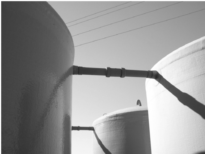
Figure 13.5. Storage tanks tied in at the top.
