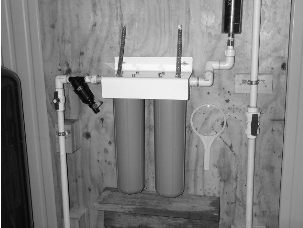
Figure 16.14. Finer filters remove particles prior to UV light exposure.
