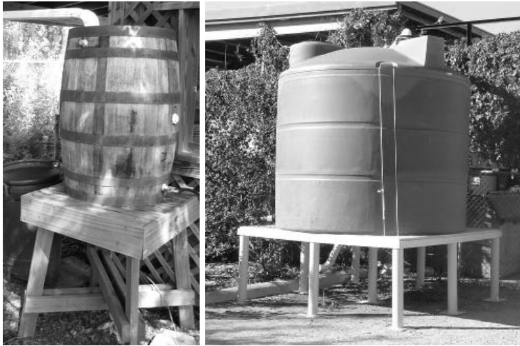
Figure 12.14. Supports for storage tanks.
