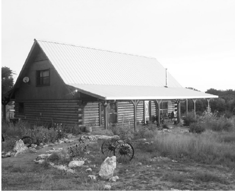
Figure 2.4. Rainwater supplies all the water needs of this home.
