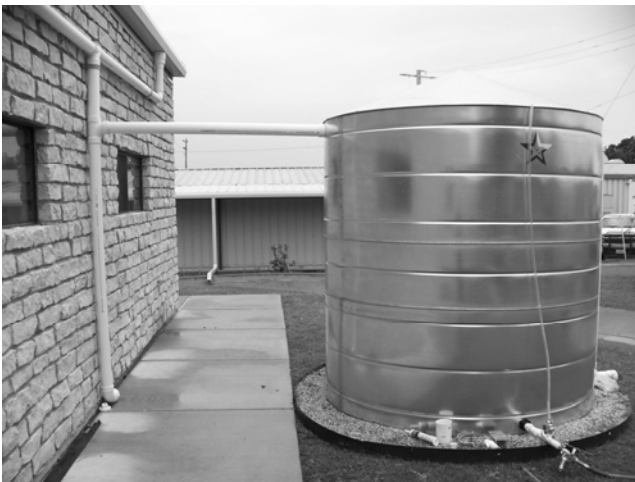
Figure 13.2. Dry conveyance can result in an overhead obstruction or an attractive nuisance for children.
