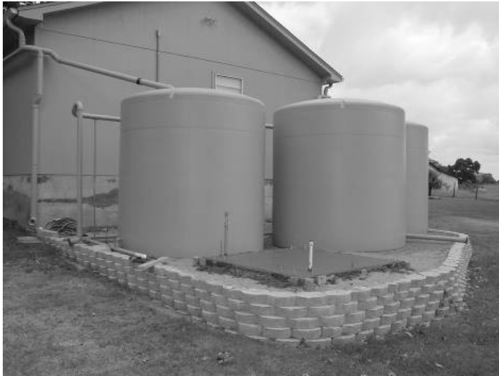
Figure 12.13. Imported soil footing for large tanks.
