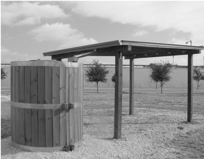
Figure 10.4. A monosloped catchment roof acts as the catchment area for the storage tank.
