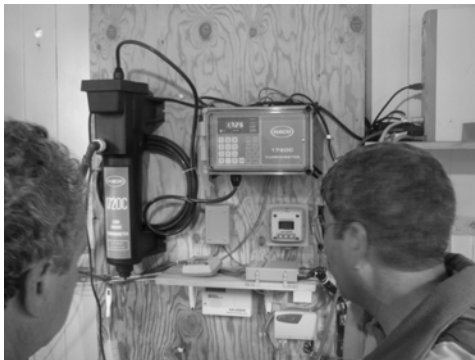
Figure 16.4. A turbidity monitor (left) ensures that water quality is sufficient to not interfere with downstream treatment measures, such as an UV light (right).
