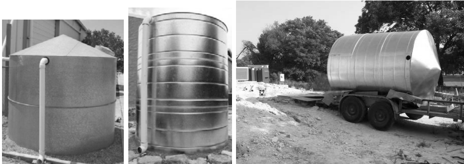
Figure 12.3. Prefabricated galvanized metal storage tanks.
