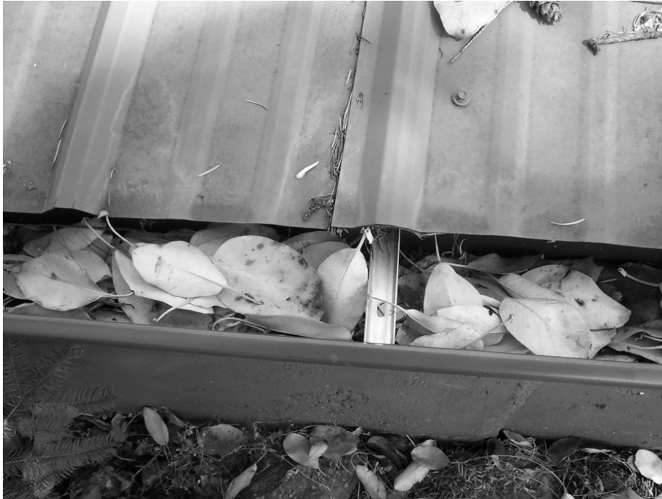
Figure 11.1. Gutters catch leaves, twigs, and other contaminants that will restrict and decrease flow of water.
