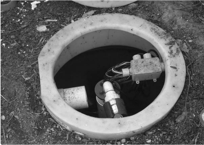
Figure 12.16. A buried storage tank is susceptible to contamination from surface runoff.
