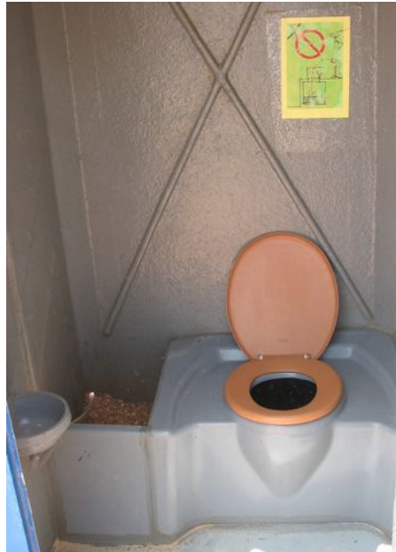
Modified chemical portable toilet housing for urine separating dry toilet, dry urinal and reservoir for wood shavings to cover feces.
