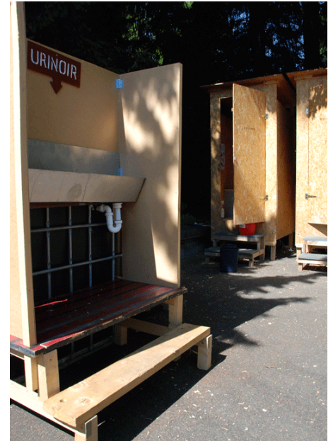
1m3 opeartes portable urinals in Geneva for bars and the City of Geneva's summer stage. The urinal drains to a 330 gallon international bulk container. Photo by Jonathan Fernandez 2010.
