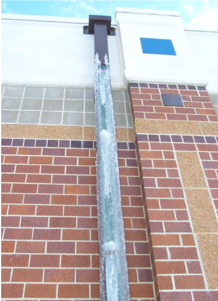
Figure 11. Accumulation of ice in downspouts draining rooftop runoff at the clay study site.
