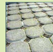
Permeable paving
