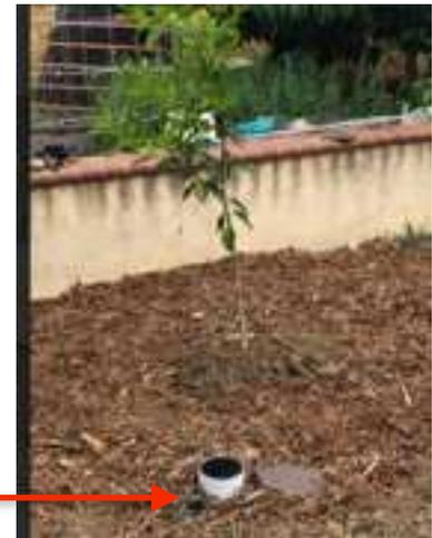
You should always see an air space underneath the graywater outlet and then wood chips below. The graywater needs to freefall out of the tubing or pipe onto mulch at the bottom of the shield to prevent roots from growing into the pipe. Soil or mulch should not accumulate so that they are in contact with the actual tubing or pipe.
